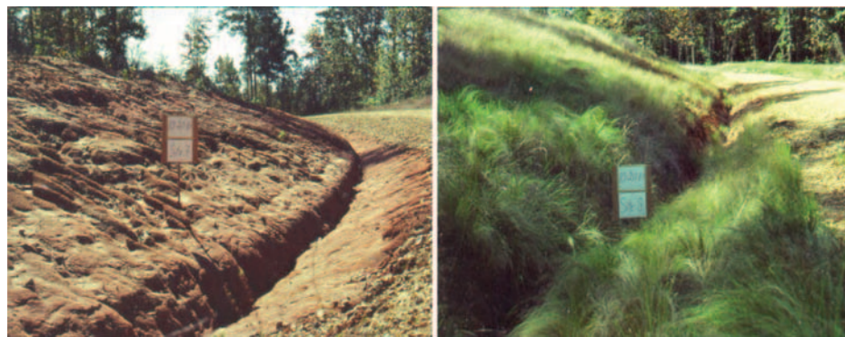
Figure 1. BMPs can dramatically reduce impacts from management activities. Here, similar forest road cuts without and with mulch and grass show the potential effectiveness of BMPs in providing cover and erosion resistance. BMPs are designed to reduce both generation and delivery of pollutants to streams and other waterbodies.
